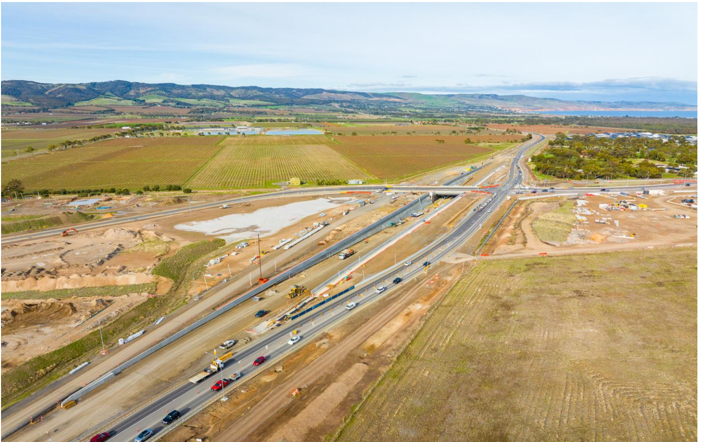
The Aldinga interchange under construction looking South
