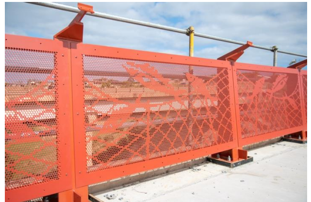
Artwork fixed to the Pedler Creek bridge, along the SUP
