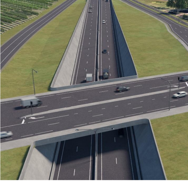
Main South Road Works
