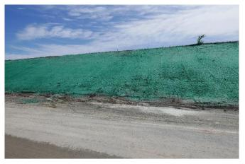
Hydroseeding is a seed planting method where seeds are combined in wet batter and sprayed onto roadside slopes.
